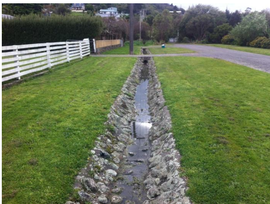
Figure 29 Lined storm water drain
